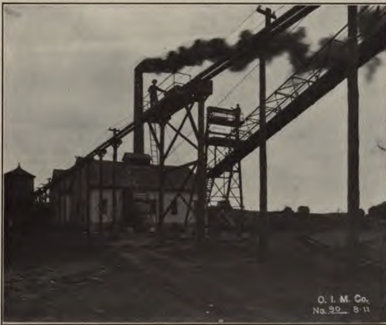
No. 13—Prince of Wales Mine, Steam Line and Idler Bridge, Negaunee, Mich.
